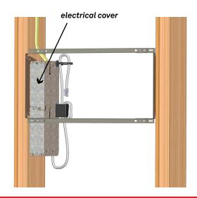
Insert cable tie mount and cable tie. Use these to support the speaker wires and other cabling that will be connected to the MS-21. Looping the PSU DC-output cable in and out of the cable tie can hold it in place temporarily until the MS-21 is ready for installation.
